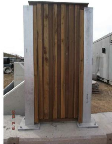
TYPICAL VIEW OF BARRIER FROM PUBLIC SIDE
